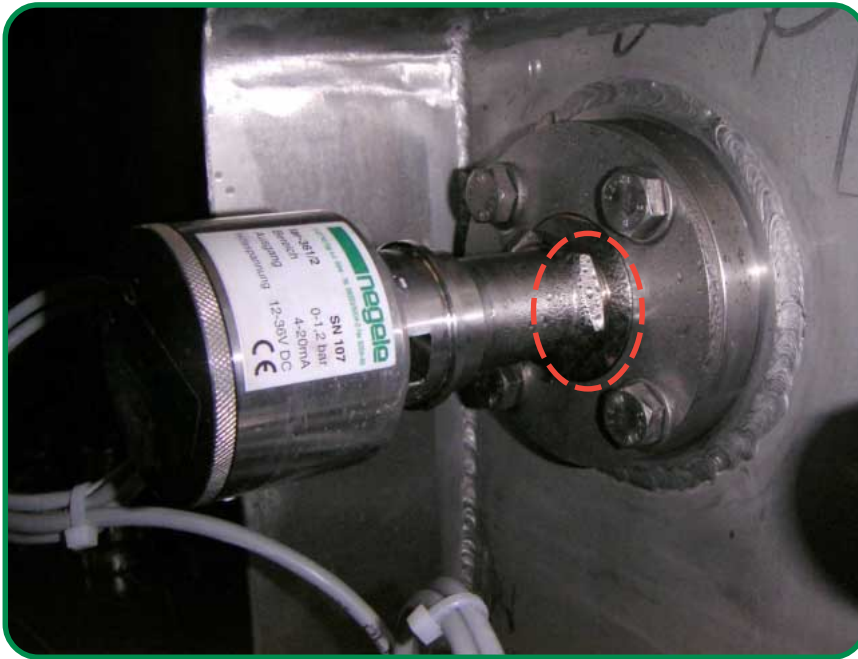
Pic.1: Condensation at the level sensor LAR-361
